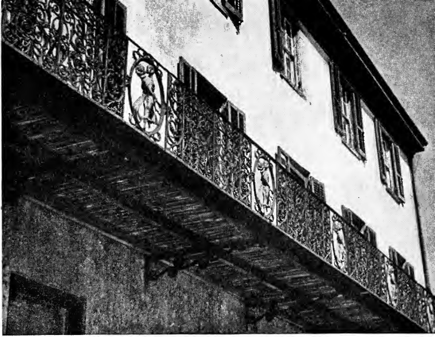
WROUGHT IRON BALCONY ON COLONIAL APARTMENTS, BORDENTOWN
